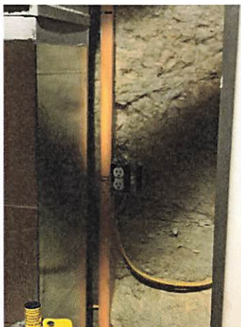
NM cable installed throughout if assembly may not be allowed.
