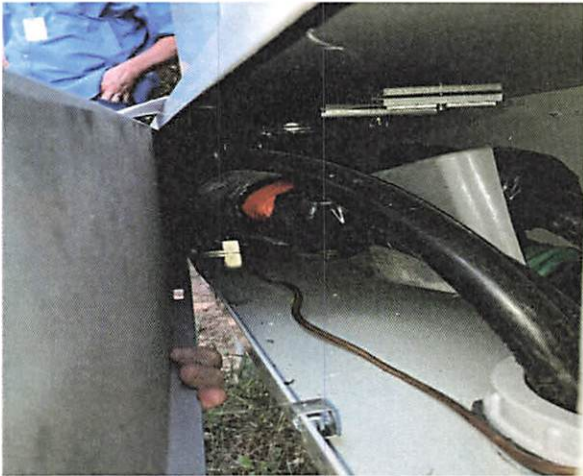
Meter enclosure only not service disconnect, unfused cable
