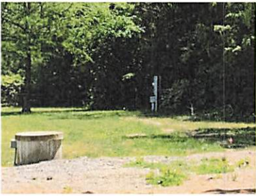
Meter enclosure only not service disconnect, unfused cable
