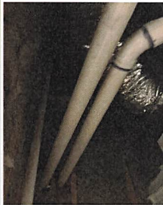
supports needed for flue vents
