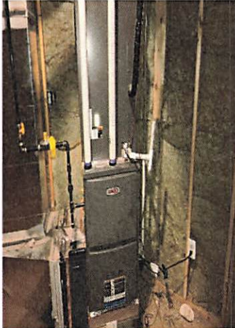
Insulation exposed paper
