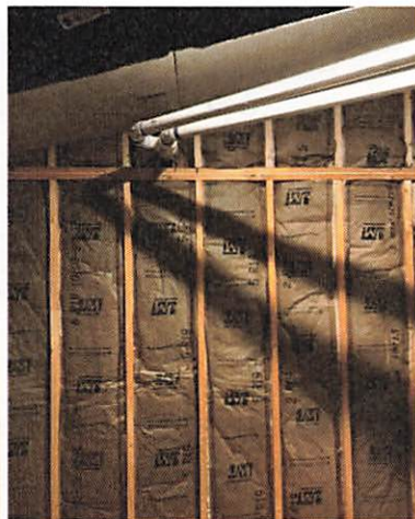
supports needed for flue vents
