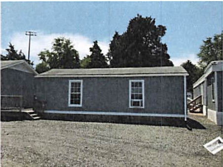
BUILDING 2 (Shed next to SFD)
