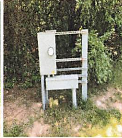
Meter enclosure only not service disconnect, unfused cable
