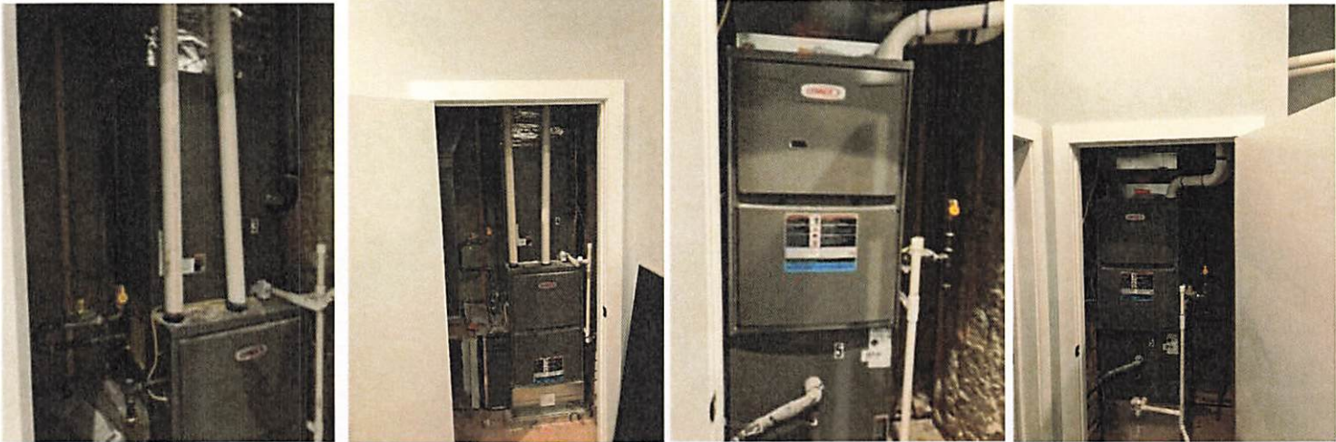
2 furnaces installed on 2 nd level above kids room
