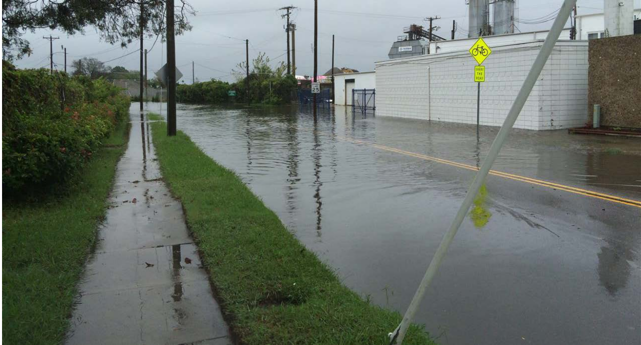
Flooding on Kimball Terrace impeding access to and from the Chesterfield Heights community. Source: City of Norfolk.
