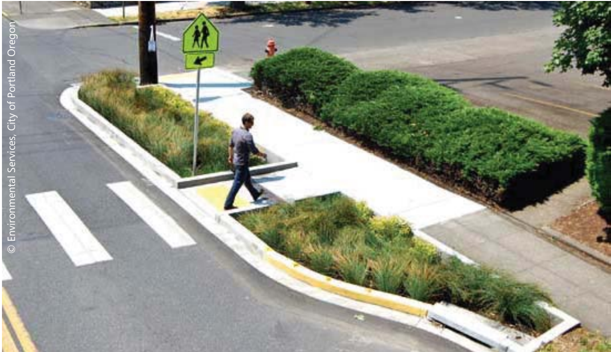
Example photograph of bioswales used as a street-wide stormwater improvement. Source: SCAPE.
