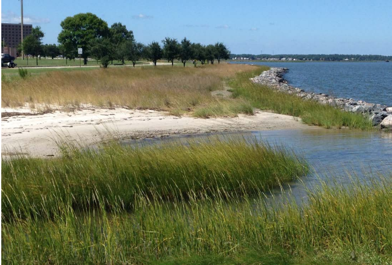
Photo illustrating a living shoreline, a design component common to all alternatives. Source: VHB.
