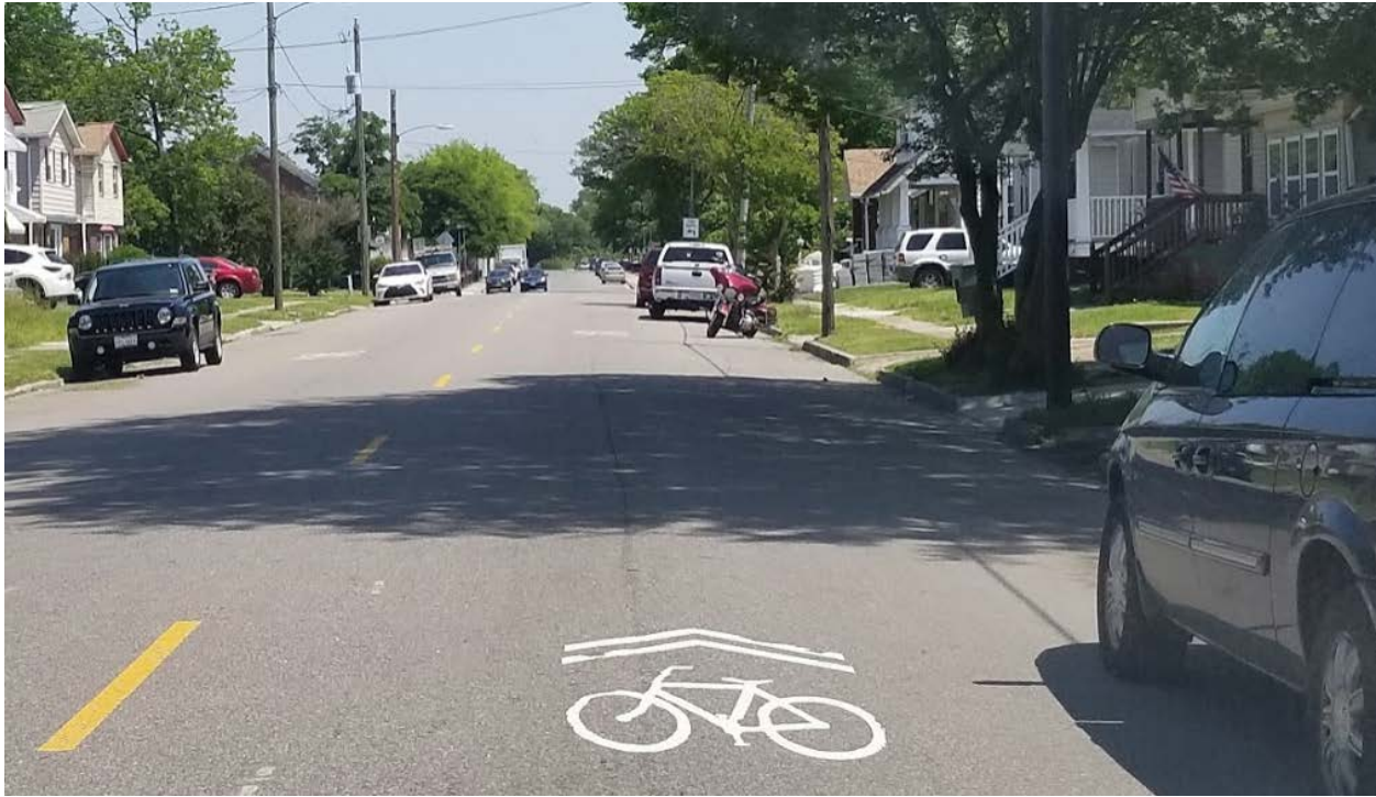
Example of a sharrow painted on Kimball Terrace. Source: VHB.
