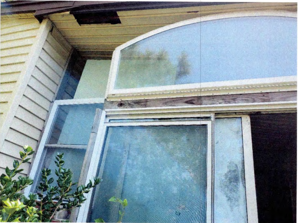
Figure 1 – Front Porch Entrance
