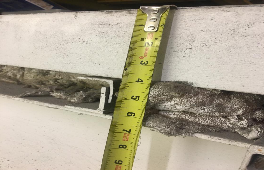
Poured Concrete Thickness
