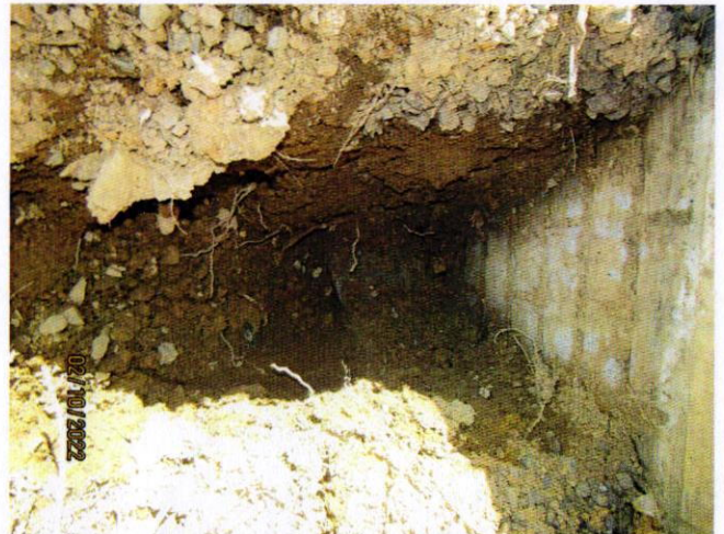
Photo 2 – Footing depth sample
