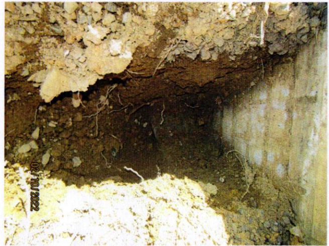
Photo 2 – Footing depth sample
