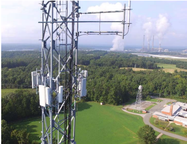
Tower Deployment in Person Co NC
