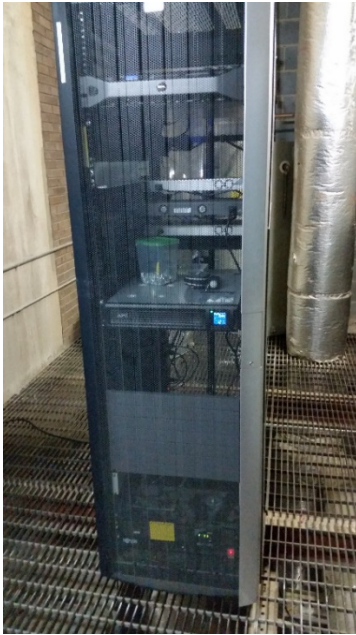
C. Secured Rack Enclosure in Air Shaft
