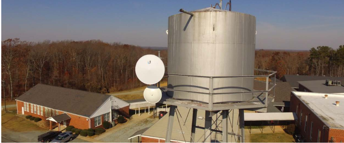
Backhaul (dual) via Water Tank
