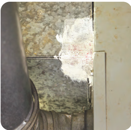
B-4. Push fiberglass mesh into the mastic
