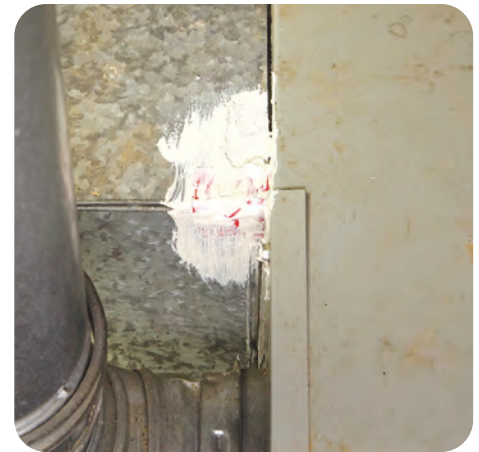
B-3. Apply mastic over the tape
