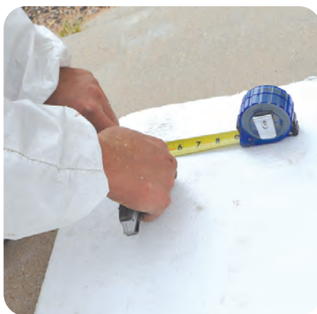
2. Cut blocking material to fit
