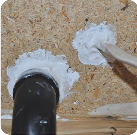
1. Ensure air sealing is complete
