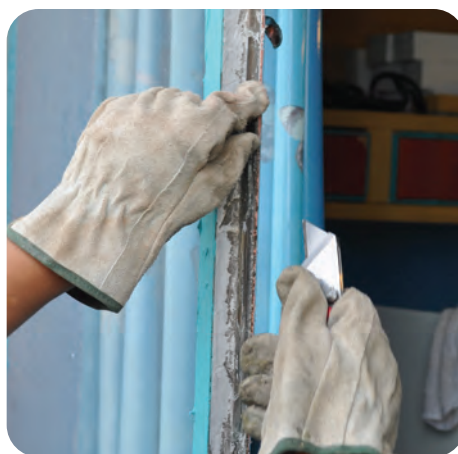
2. Clean all debris, caulk, etc., from sash
