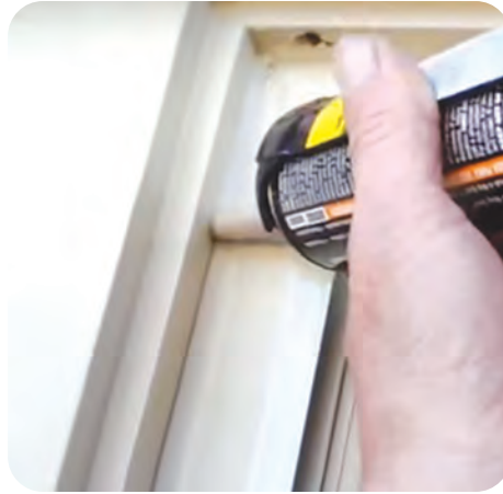
8. Caulk all exterior edges
