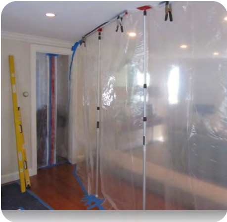
1. Protect work area from debris and dust
