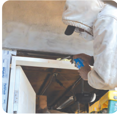
8. Insulate gaps between door jamb and frame
