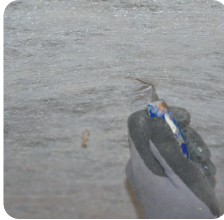
12. Cut access hole for fill tube
