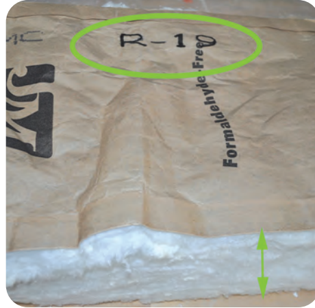
2. Insulation R-value matches work order
