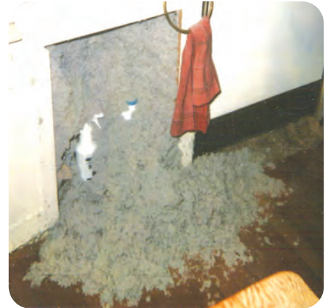
3. Ensure wall integrity is complete (no holes)
