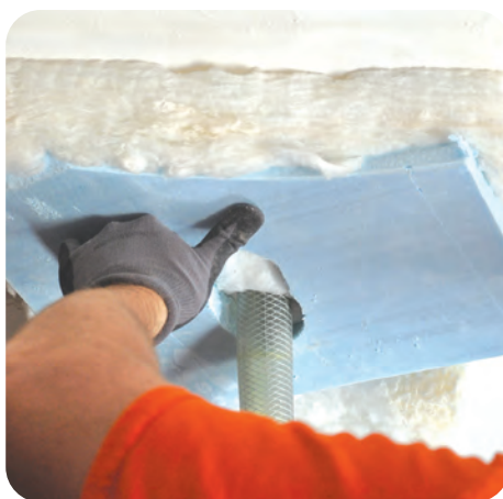
6. Blow insulation to completely fill cavities to prescribed density
