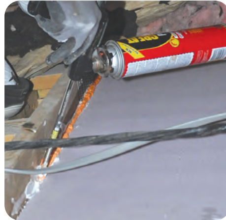
B-2. Seal around infill materials
